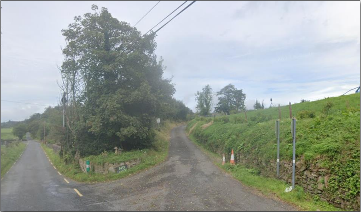
Figure 6 WDA Access Road
